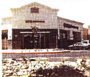
Regency Center's Jefferson Square shopping center in La Quinta, Calif., has achieved LEED Gold certification from the USGBC.
